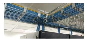
**PROPATCH** Mesh Basket Trays, Ladder Tray etc. LCP can Supply length and Width according (Available in different Sizes) to customers request.
